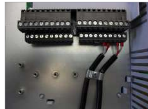
(b) Connection sample of the shield to ground
