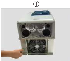
Removal of the fan grid screws
